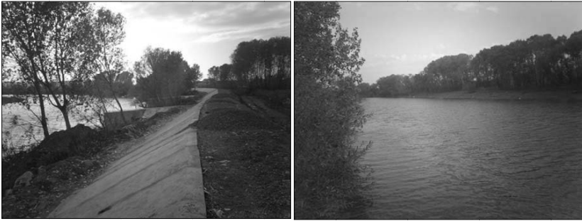
Figure 5-9: Enforced embankment and the opposite side
